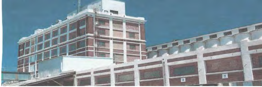
The 1917 flour mill, an 8 story tower + 2 story building, with silos behind. Designed by Maurice C. Couchot, and celebrating its centenary next year.
