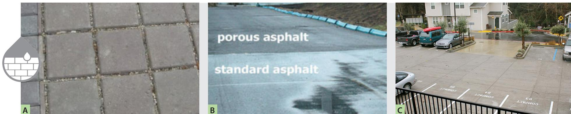
**A. Permeable pavers at UC Berkeley Botanical Garden (source: Blue Green Blog, Friends of Five Creeks) B. Pervious asphalt comparison (source: Water Research Center) C. Residential parking lot with pervious concrete (source: Fall Creek Engineering, Inc.)**
