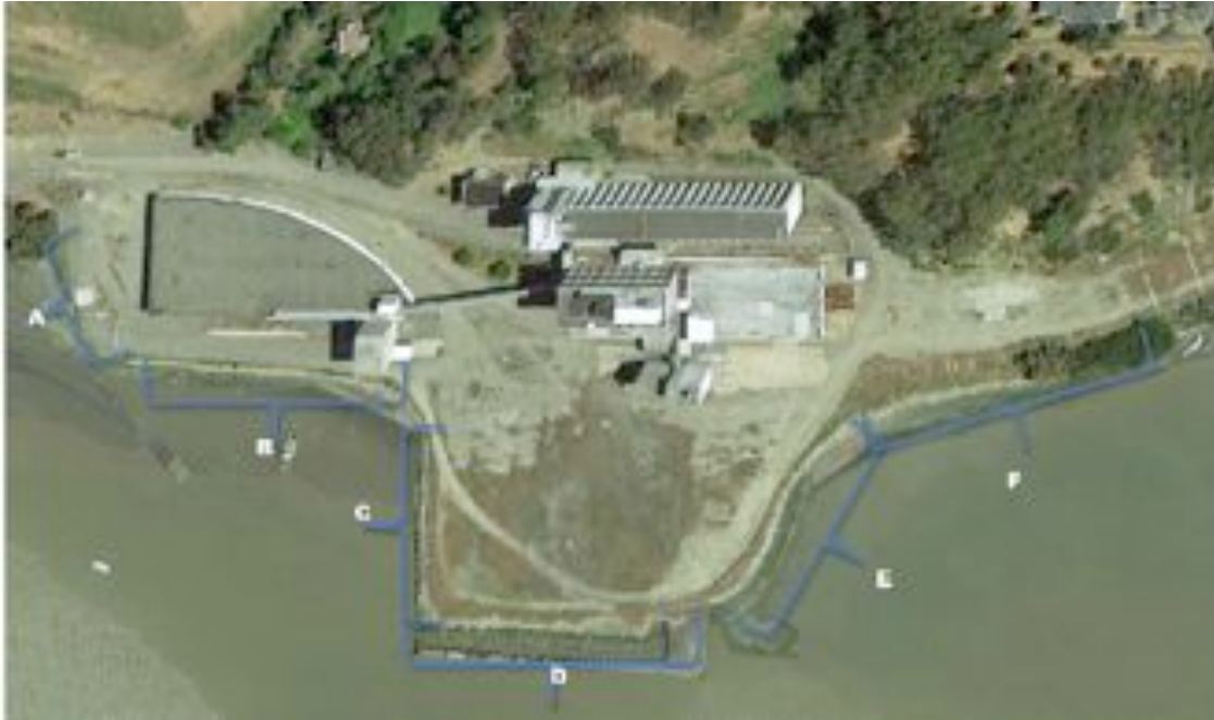
Figure 2-1. Vallejo Marine Terminal survey site locations.
