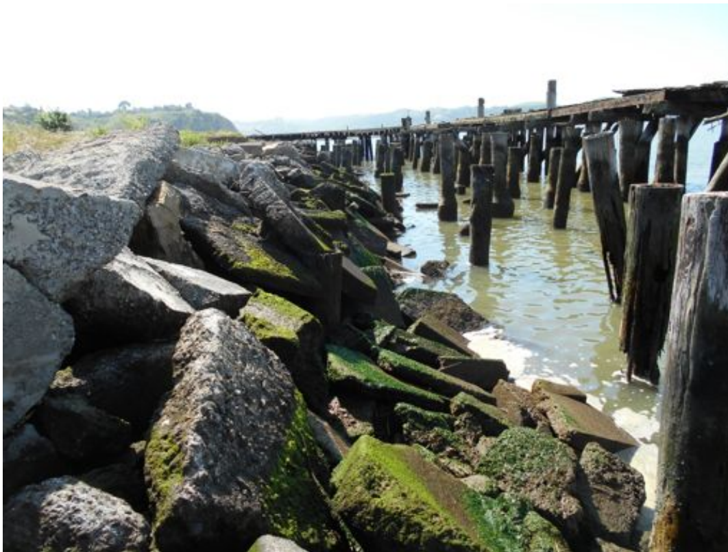
Figure 3-1 Survey Segment D, Concrete Slab Bulkhead. The light green algae is the filamentous form of Ulva spp. and the dark green is the leafy form of Ulva spp.
