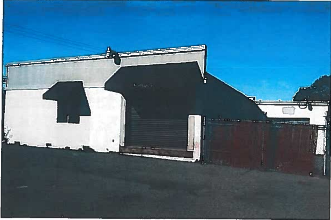
Figure 7 South and East Elevations; View to the Northwest
