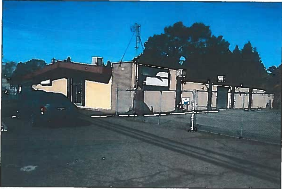
Figure 8 South and East Elevations; View to the Northwest
