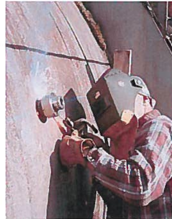
Hot-tap transducer installation
