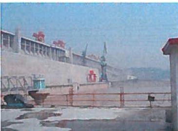
View of the Three Gorges Dam tailrace from the Right Bank entrance.
