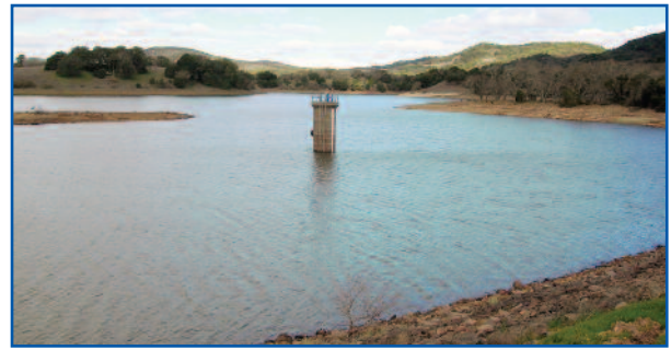
Lake Madigan Source Water for the Lakes Service Area
