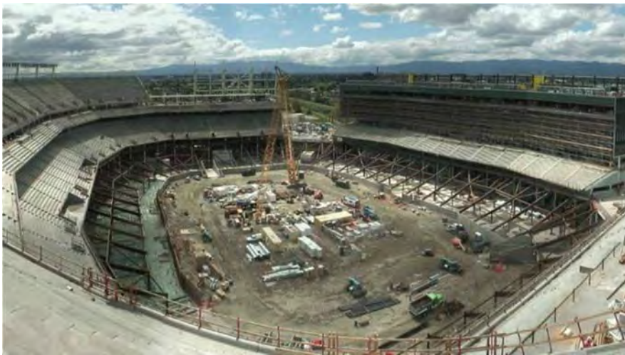
Figure 6: New 49ers Stadium in Santa Clara
