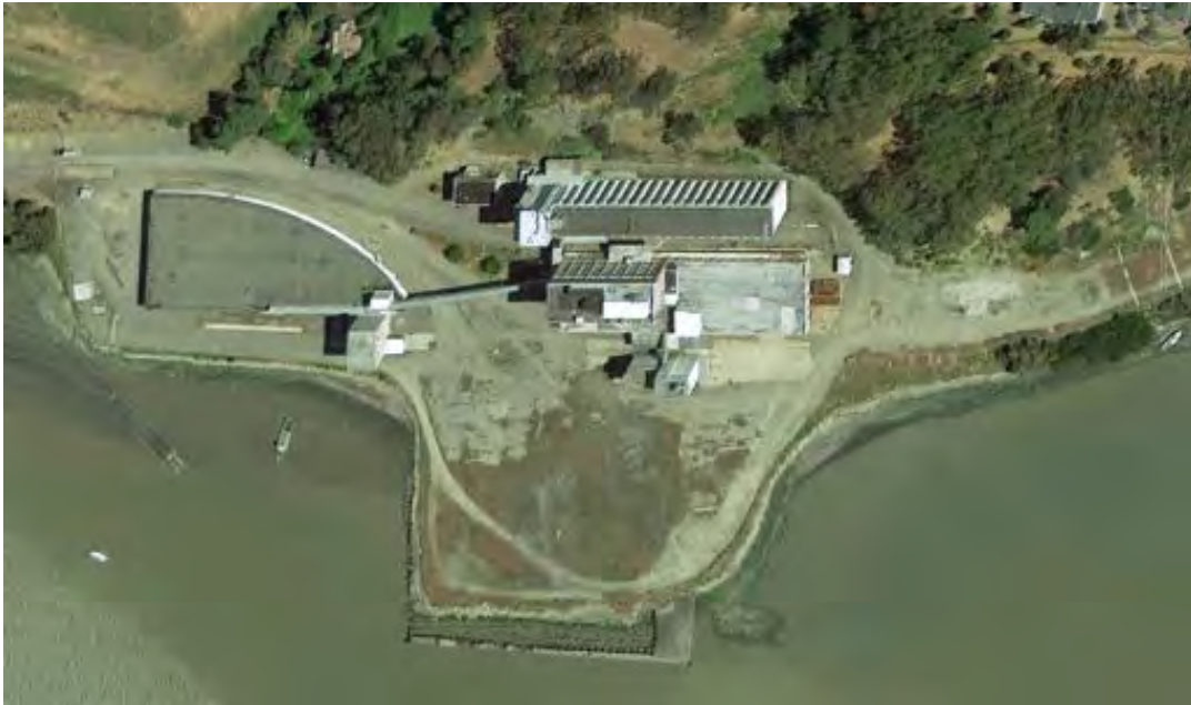
Figure 1-1. Existing shoreline conditions and intertidal habitats along the Vallejo Marine Terminal Site waterfront, Vallejo, California.
