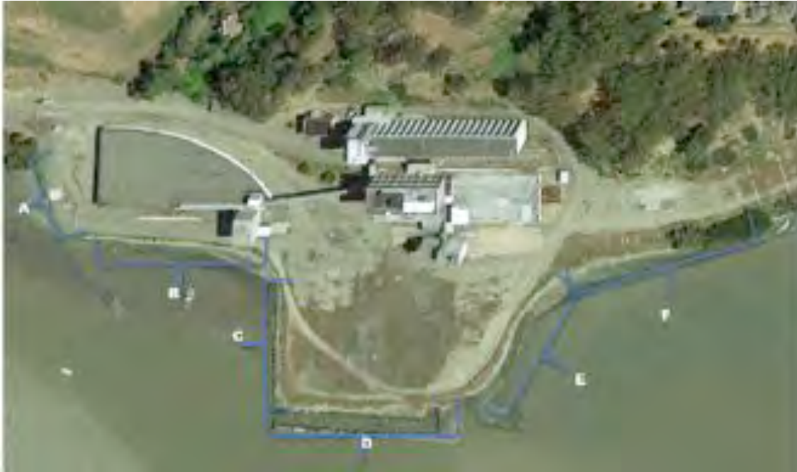
Figure 2-1. Vallejo Marine Terminal survey site locations.
