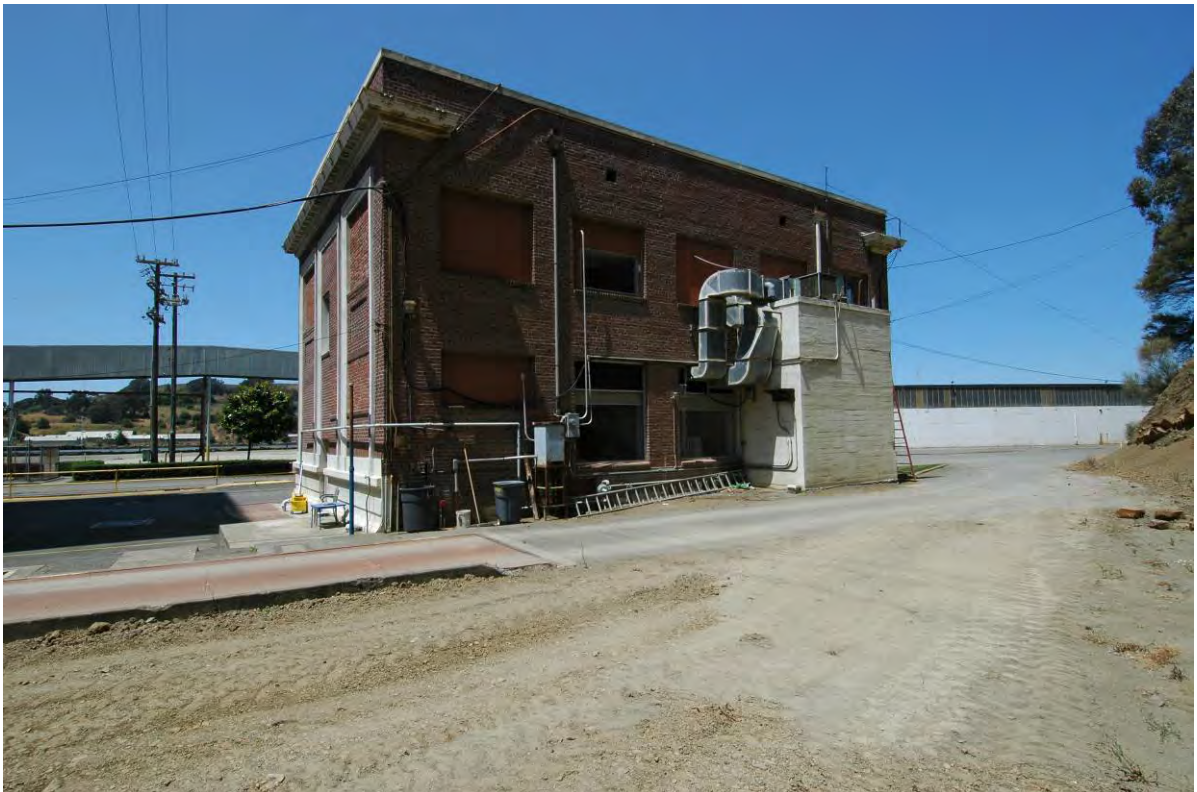
Administration building, rear elevation. Carey & Co., Inc., 2007.
