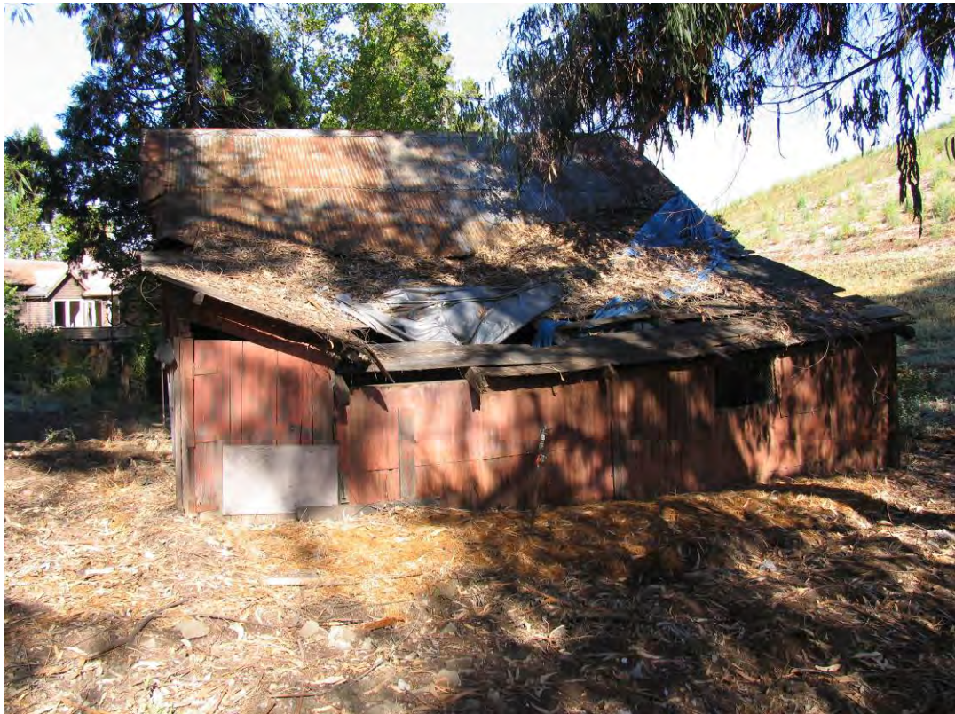
Barn, east elevation. Carey & Co., Inc., 2007.
