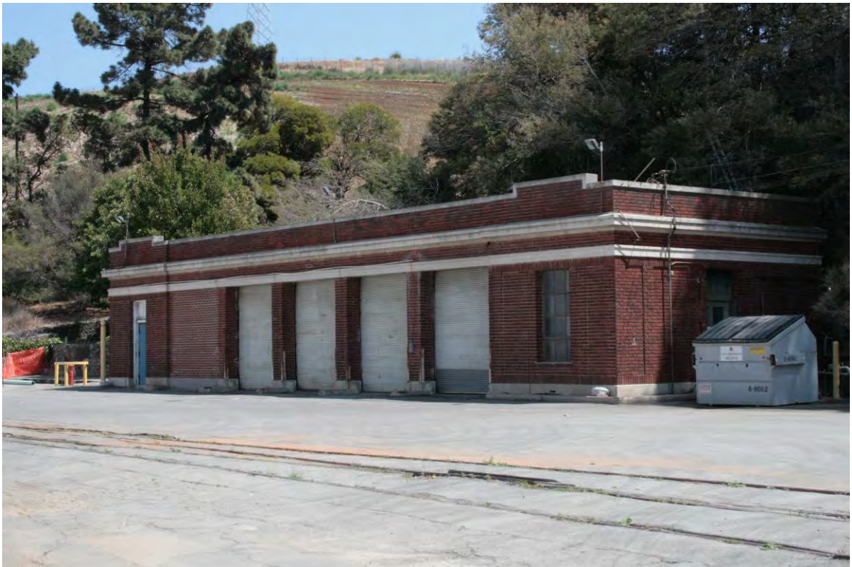
Plant garage. Carey & Co., Inc., 2007
