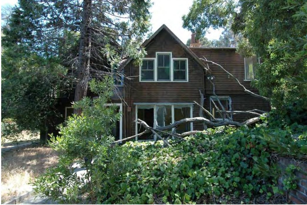
Manager's House, front (west) elevation. 1917 additions to left and right of central gable. Carey & Co., Inc. 2007.
