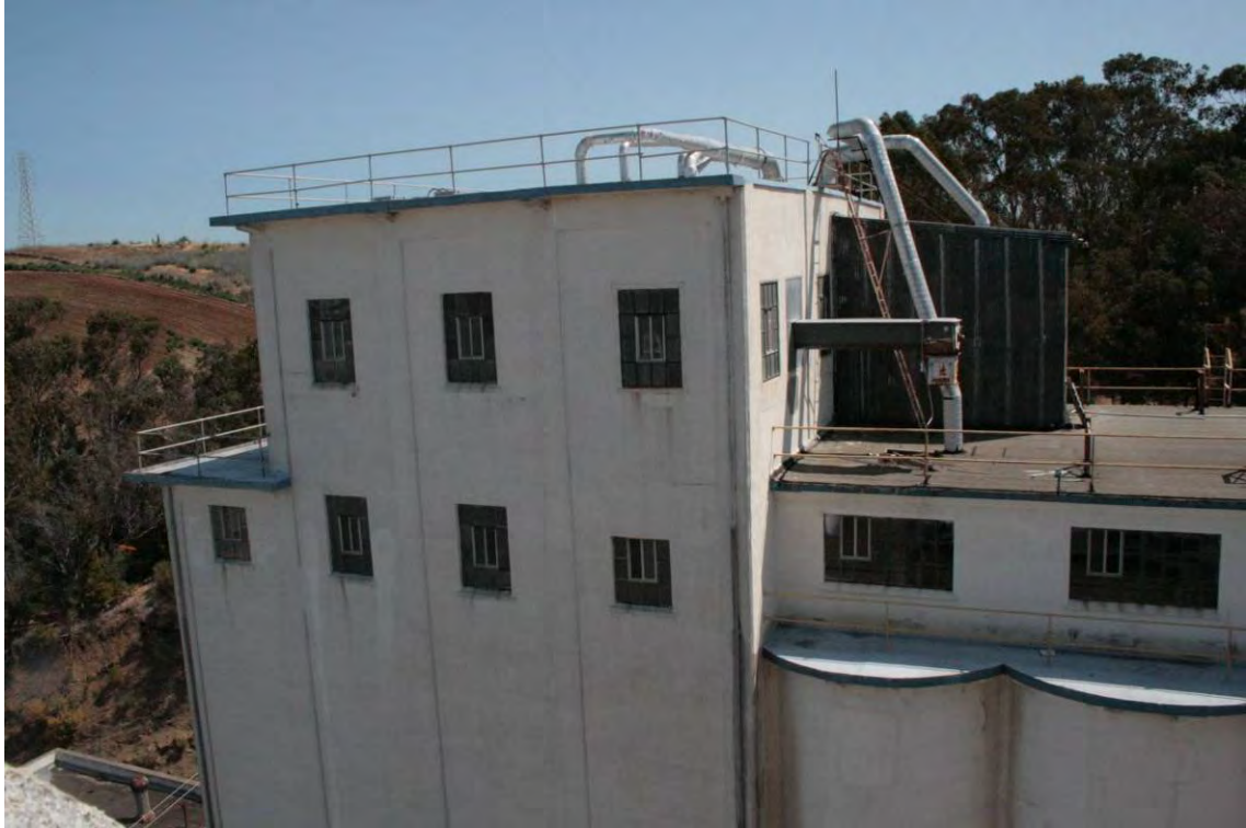
Head house, grain elevator. Carey & Co., Inc., 2007.
