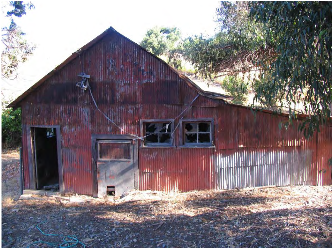
Barn, south elevation. Carey & Co., Inc., 2007.
