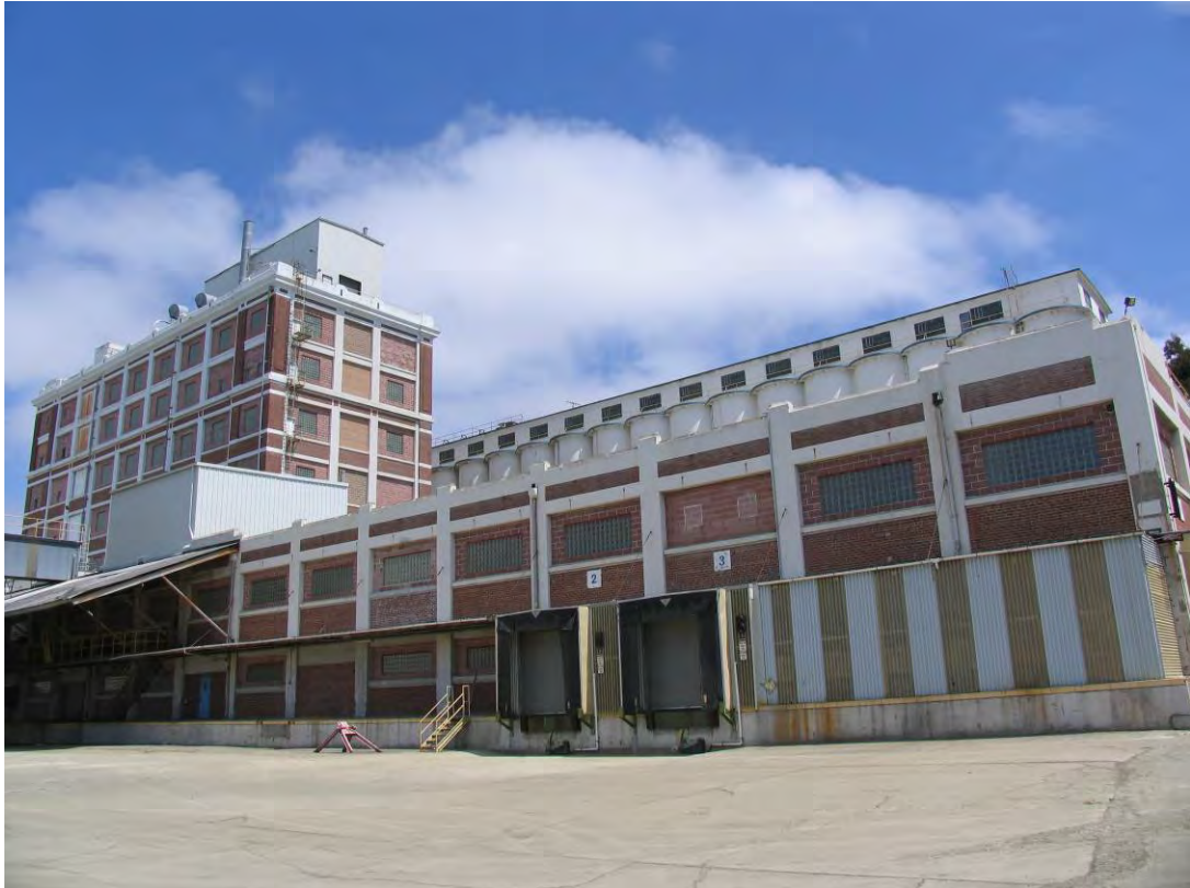
Flour mill and warehouse with top of silos in background. Carey & Co., Inc., 2007.
