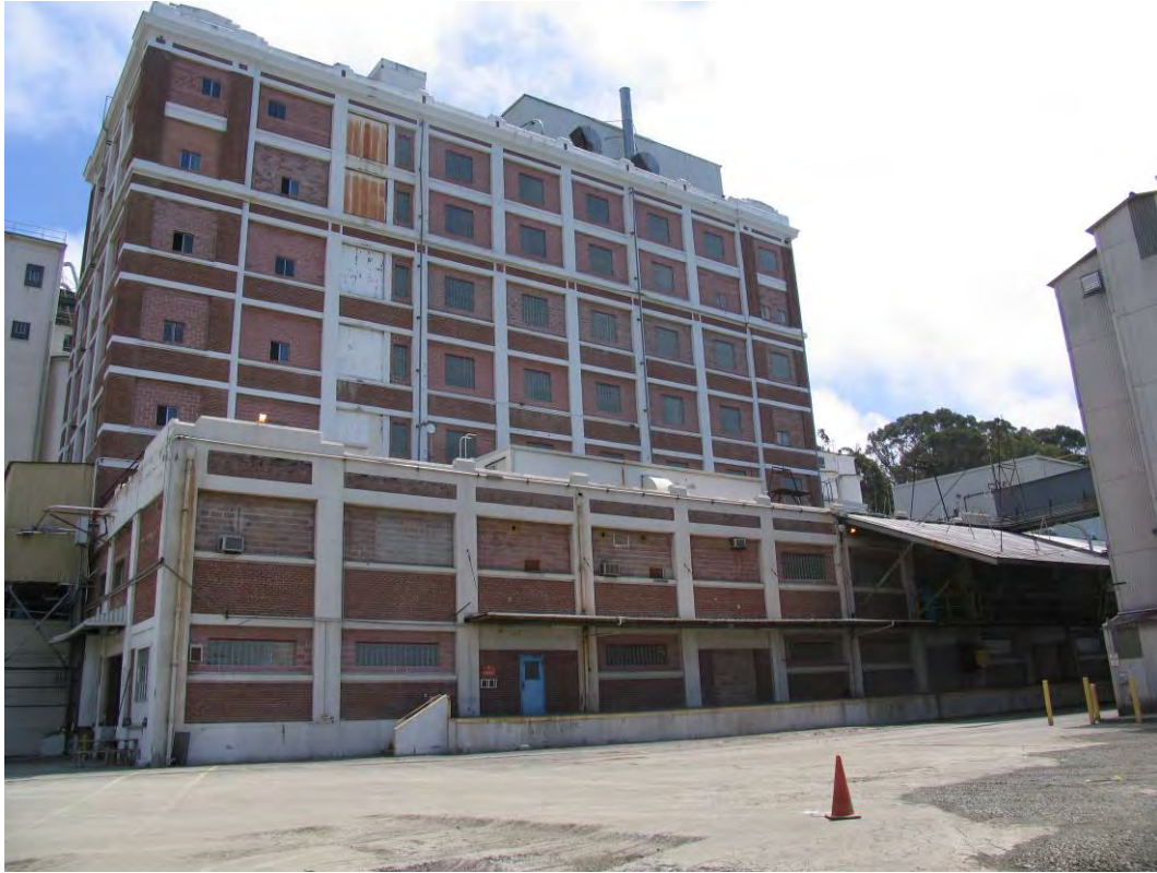
Flour mill and warehouse, west elevation. Carey & Co., Inc., 2007.
