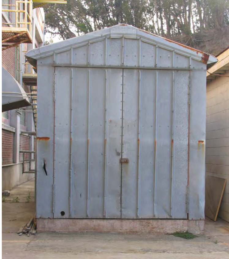
Welding shop. Carey & Co., Inc., 2007.
