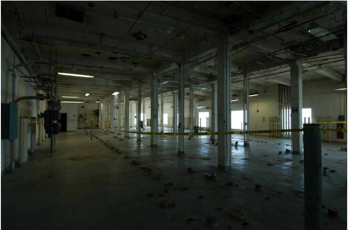
Mill, interior. One of the processing floors. Carey & Co. Inc., 2007.
