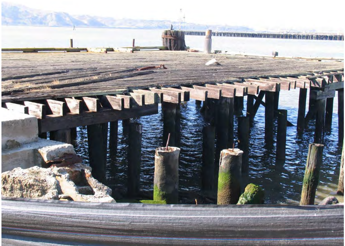
Dock with traces of railroad tracks. Carey & Co., Inc., 2007.
