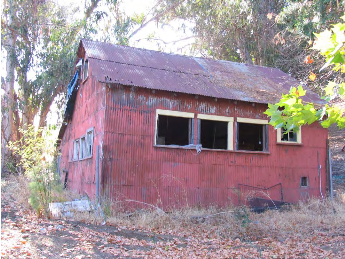
Barn, west elevation. Carey & Co., Inc., 2007.
