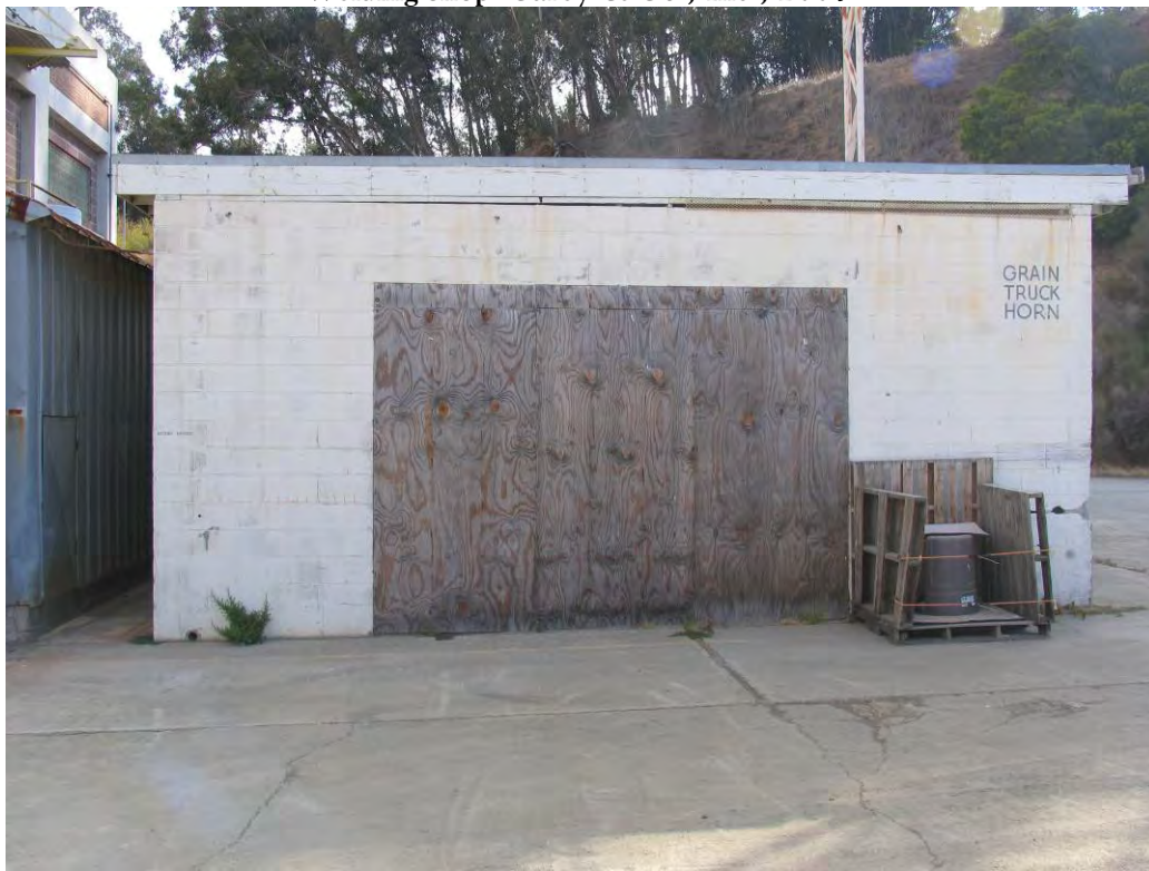
Pipe Storage. Carey & Co., Inc., 2007.
