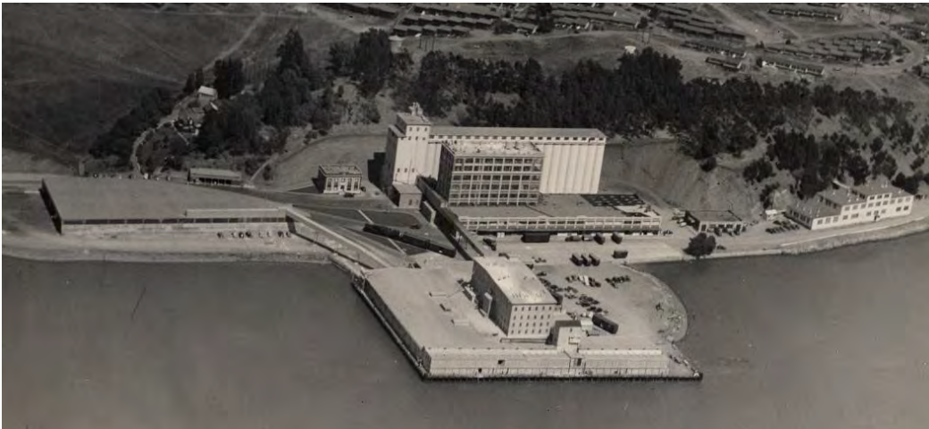
General Mills, Vallejo plant, c. 1947. The old Starr Mill stands near the bottom of the photo, while the new feed warehouse is located at the far left and the bag factory is located at the far right. Courtesy of Floyd Miller and the Quarter Century Club, General Mills.
