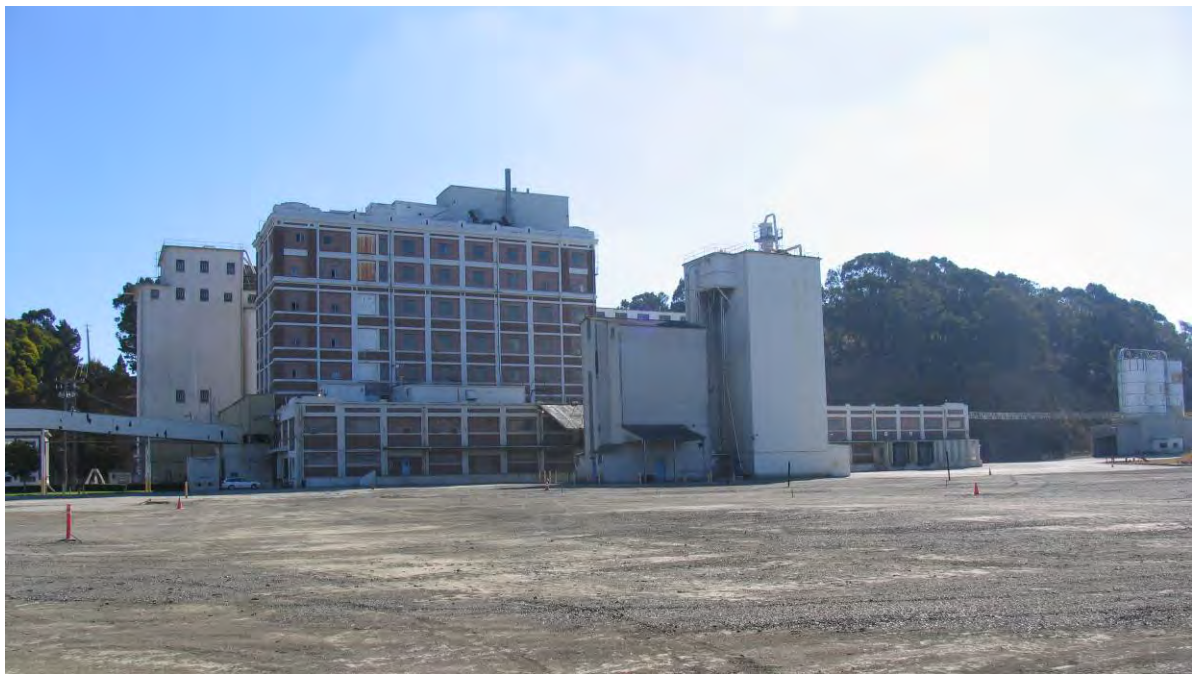
View from dock. Carey & Co., Inc., 2007.
