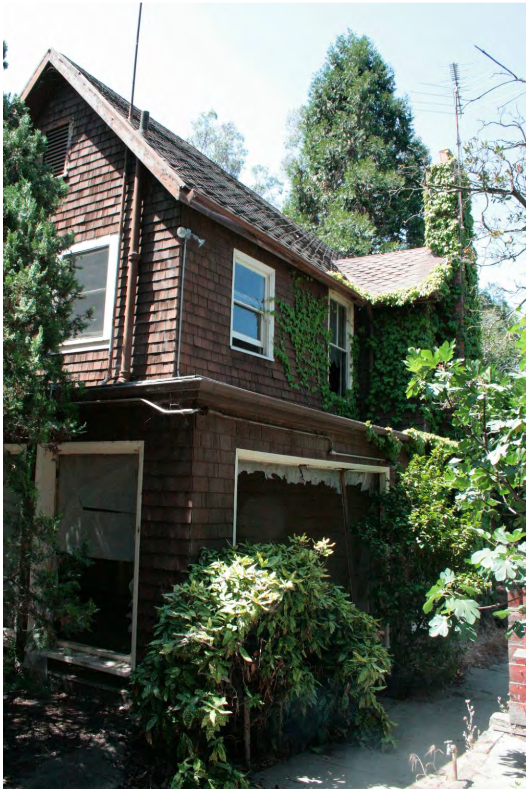
Manager's House, side (northeast) elevation showing 1919-1951 alteration to first story. Carey & Co., Inc., 2007.
