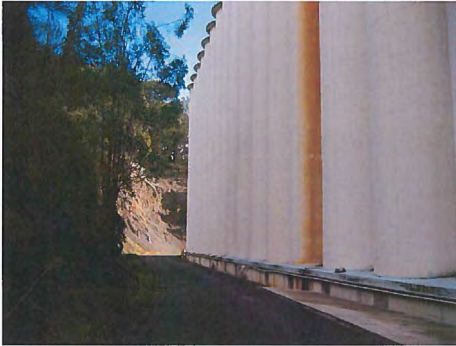
15. Eastern side of Grain Elevator building and drainage area, view to the southeast.
