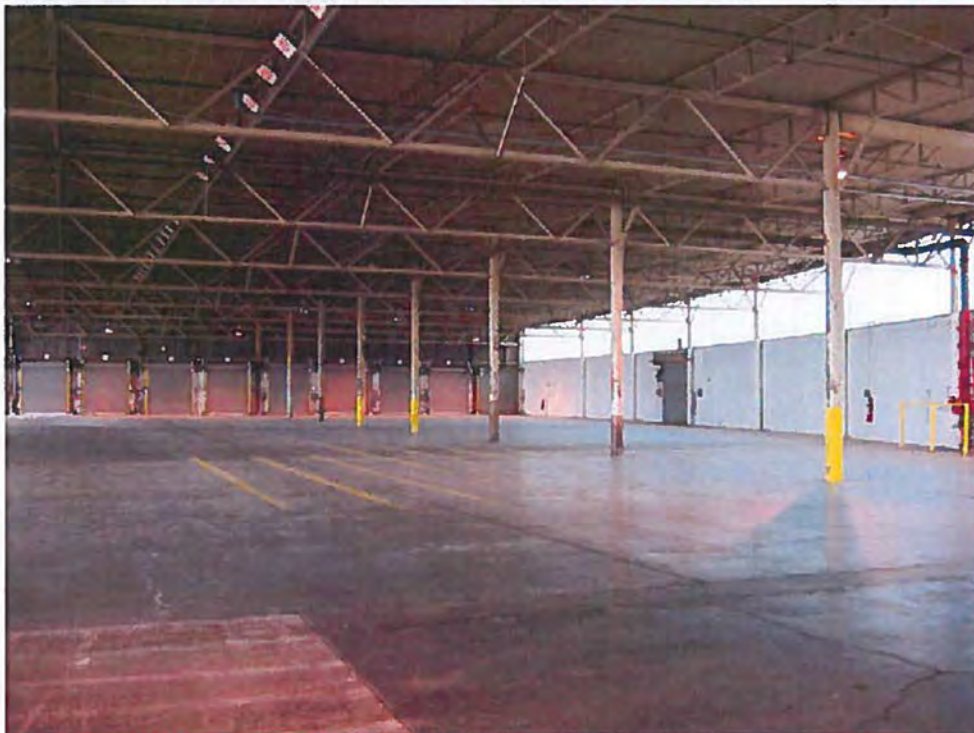
12. Interior of New Warehouse building.
