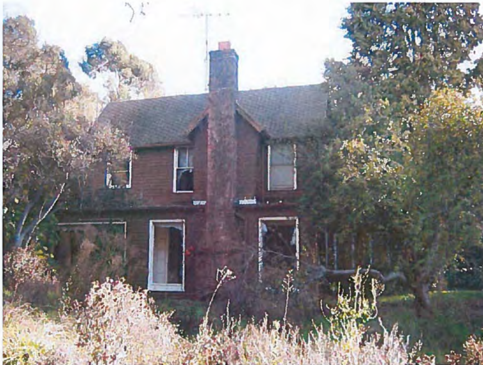
9. Plant residence, view to the east.
