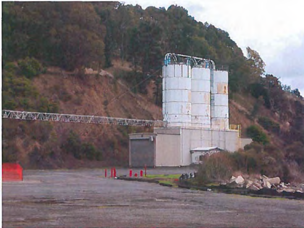
5. Mill run building on southern portion of the Site, view to southeast
