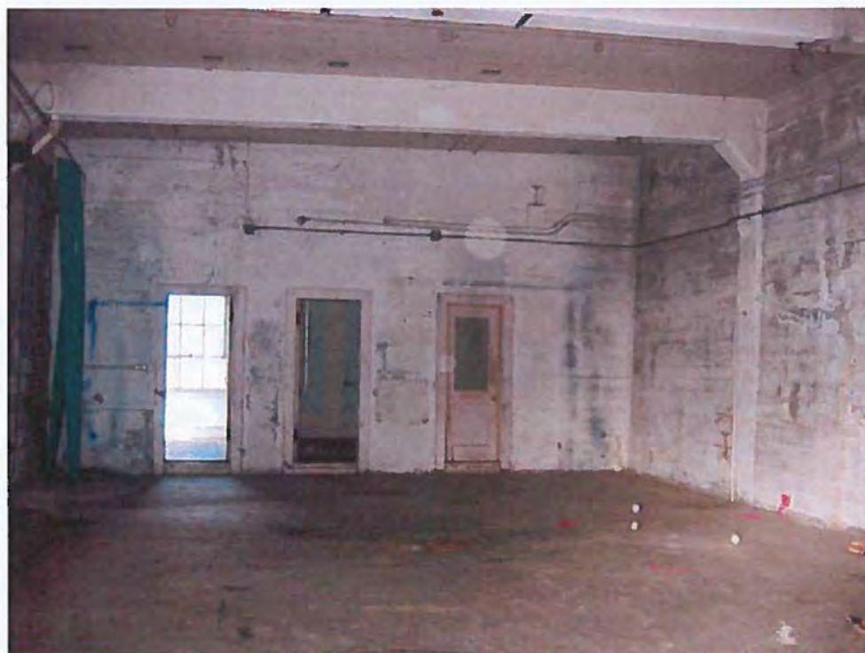
8. Interior of Garage building.
