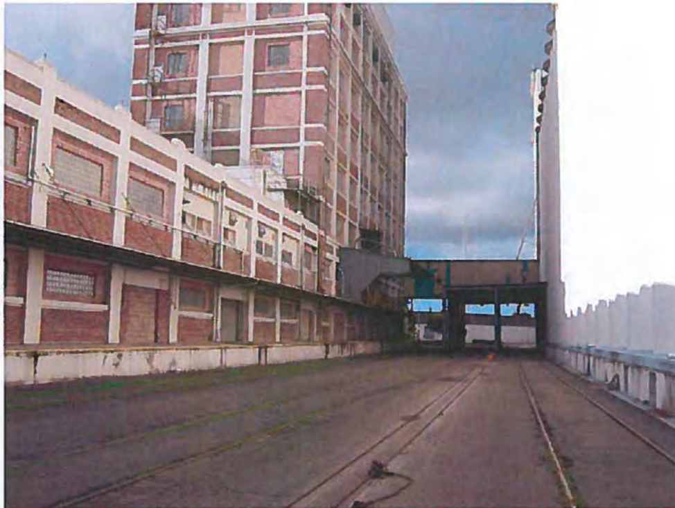
19. Railroad spur between Grain Elevator Building and Old Warehouse and Mill building, view to the northwest.
