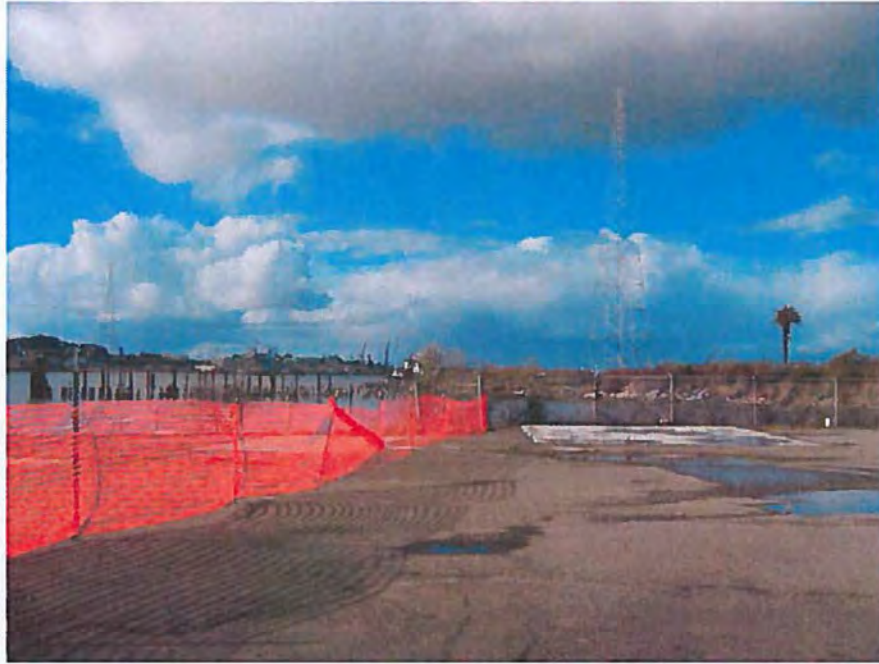
13. Former UST area T-1, T-3, T-4, and former AST area AST-4 and AST-5, northwest of the New Warehouse building, view to the northwest.
