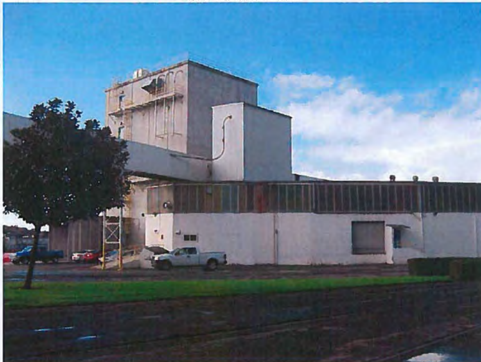
20. New Warehouse building and Truck Loading Building, view to the west.
